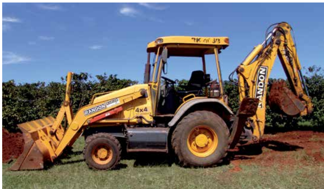
Figure 1. Backhoe for construction of the trenches.
