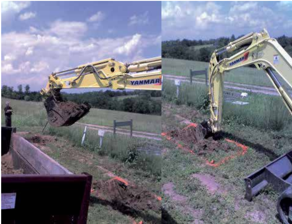
Figure 7. Preparation of soil cavity for biofilter installation at Kentucky State University (Franklin Connty, KY) for trapping herbicides residues in surface runoff water.
