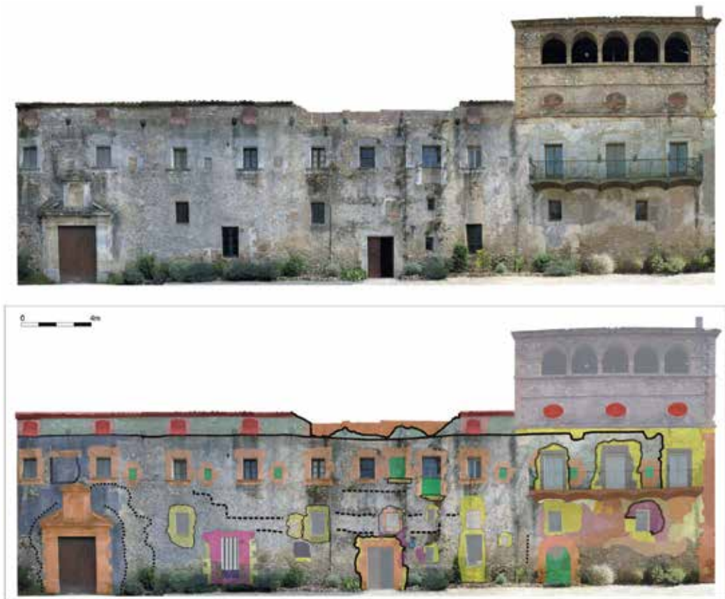
Fig. 8. Orthoimage of the main façade from the Castle of Penyafort (Catalonia) with the SU registers representation.
