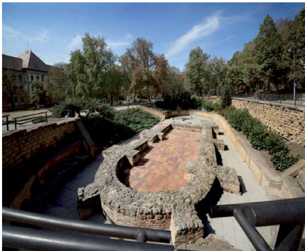
Fig. 6. The ground walls of the Early Christian Mausoleum
