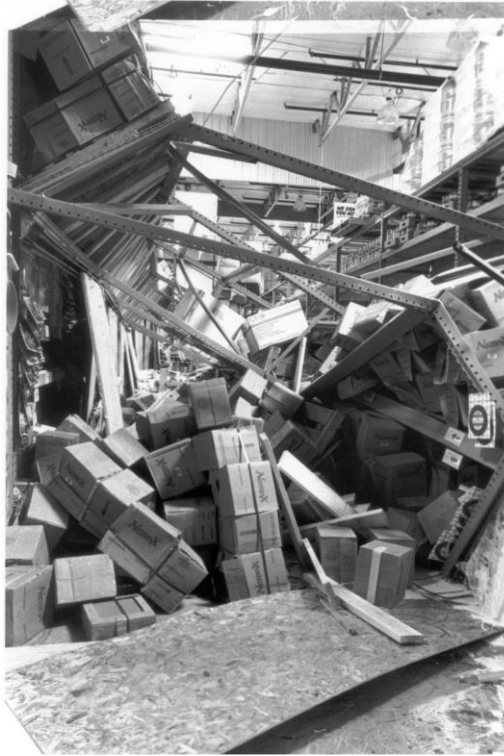
Figure 1. Damage to overloaded racks during the 1994 Northridge (USA) earthquake (FEMA E-74, 2012)
