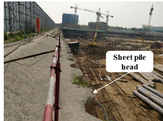
(b) Sheet piles of retaining structure
