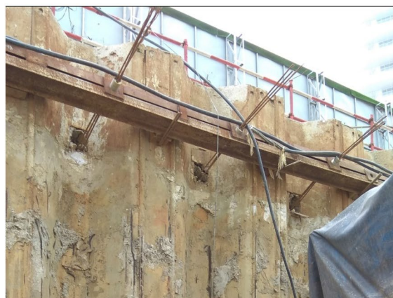
(c) Installed anchors
