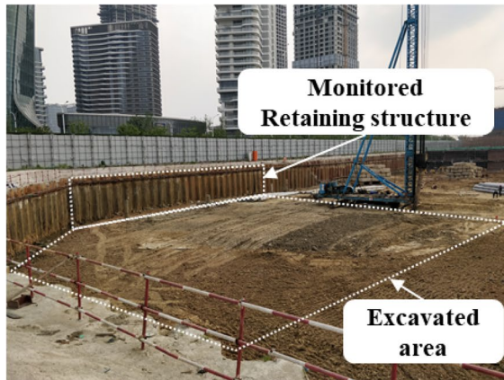
(a) Excavation site
