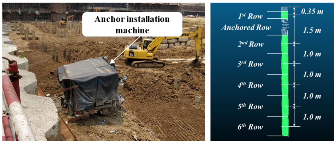
(b) Shadowed area due to anchor installation (c) Divided element in a sheet pile
