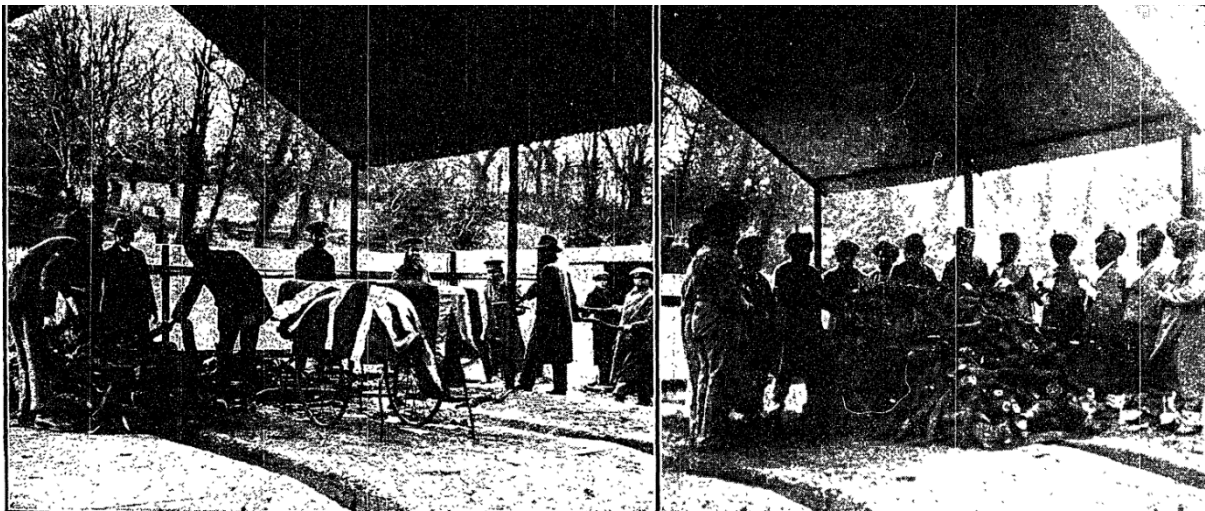
Figure 21. Two photographs published in the Manchester Guardian of the preparations for the funeral of a Hindu Indian serviceman who died at the Royal Victoria Hospital, Netley, in February 1915. In the left image volunteers of the Indian Ambulance Corps construct the deceased's pyre, whilst his coffin awaits cremation. In the image to the right sepoy patients have arrived to participate in the ceremony. 74
