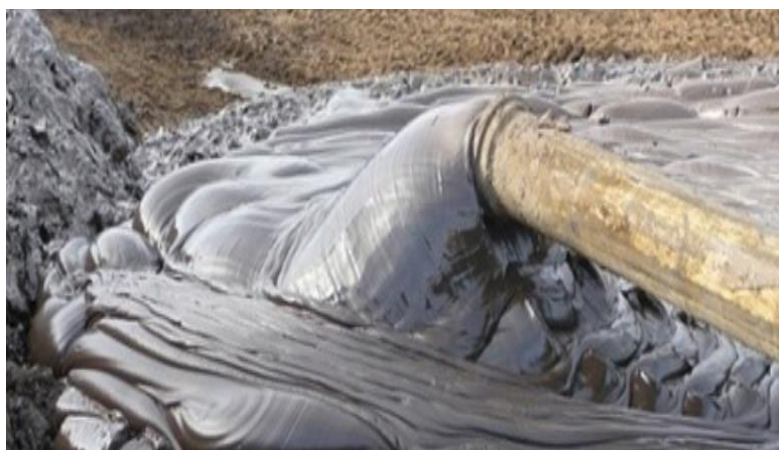
Fig. 2.6 Paste fill discharge (source: benp.com)
