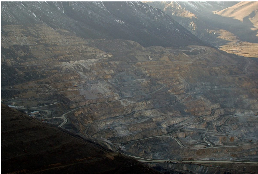
View of the Kajaran Copper-Molybdenum open-pit mine in Armenia's southern province of Syunik. Photo credit: Serouj (Courtesy of Hrayr Savzyan) – Own work, CC BY 3.0
