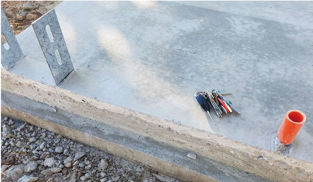
Figure C.2. Edge of concrete slab prior to framing erection
