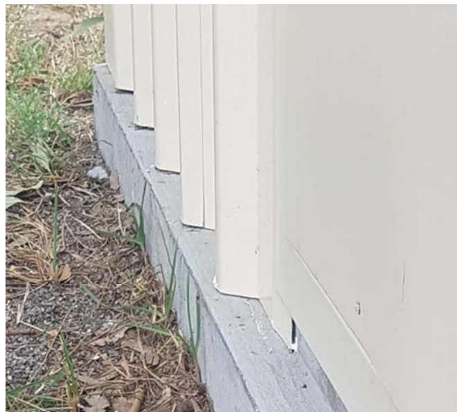
Figure C.3. JCU-ASIS wall cladding adjacent to slab rebate
