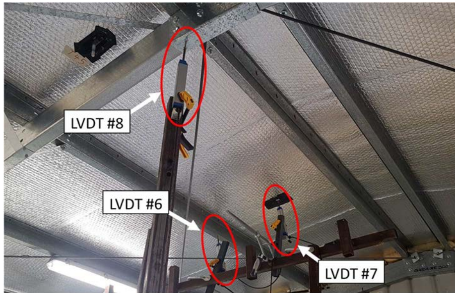
Figure 4.21. LVDT #6, #7, and #8, mounted on the roof cladding and purlin perpendicular to the roof slope, and vertically at the central portal frame apex gusset plate
