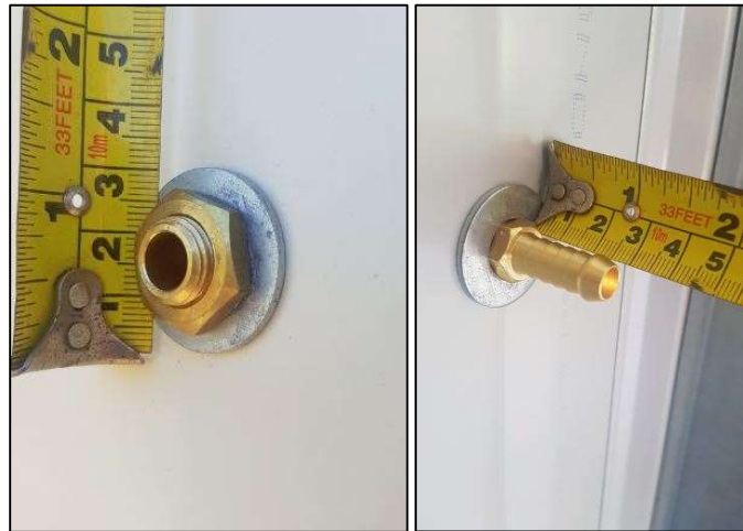
Figure 4.7. Un-instrumented pressure tap from building exterior (left) and interior (right)
