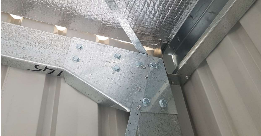
Figure C.4. Bolted gusset plate – Knee connection
