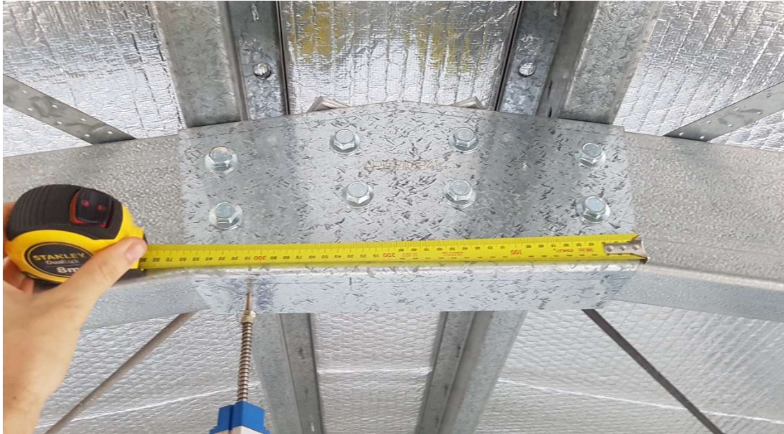
Figure C.5. Bolted gusset plate – Ridge connection
