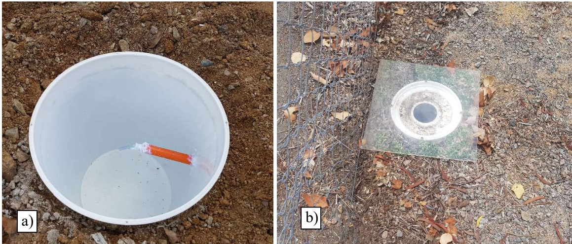
Figure B.6. FSTE reference pressure pit (a) Installation of underground tubing/conduit into pit (b) Pit in situ with flat Perspex lid
