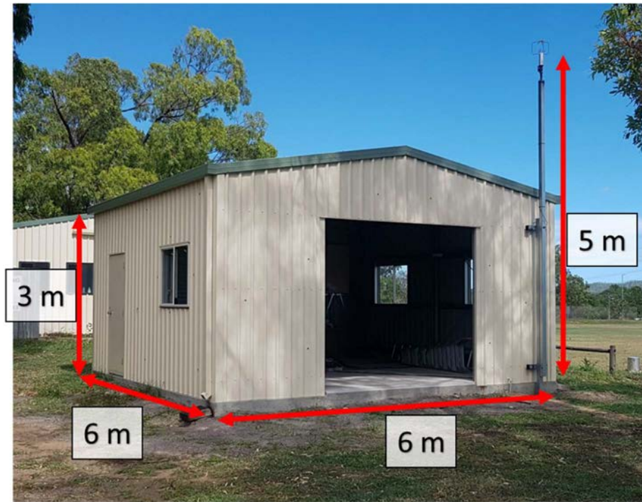
Figure 4.2. James Cook University – Australian Steel Institute Shed (JCU-ASIS) with roller door open on Eastern Wall. Sonic anemometer attached to 5 m mast at NE edge
