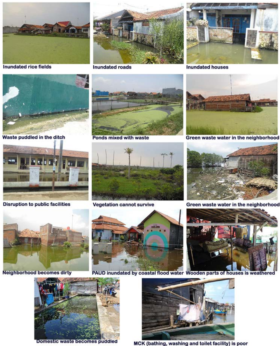
Figure 3. Impacts of tidal floods in Pekalongan coastal areas
