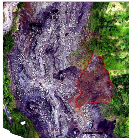
Figure 7. Aerial photo of riverbank failure (delineated by the red line) in some parts of the Gendol river valley. This location is close to the research area, located 200 m from point J in Figure 4.
