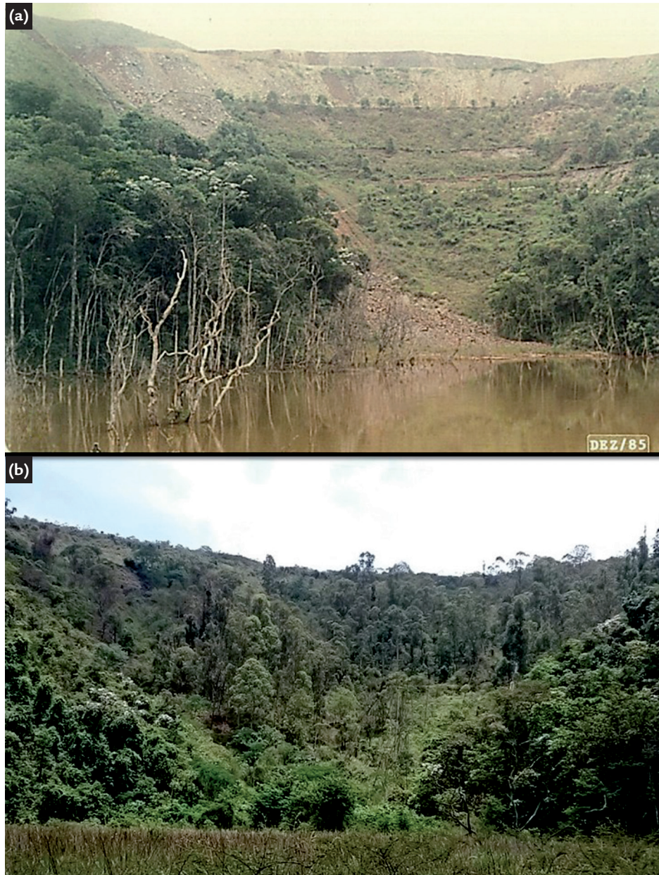
Figure 1 The waste rock dump during the construction phase (a) and current (b).
