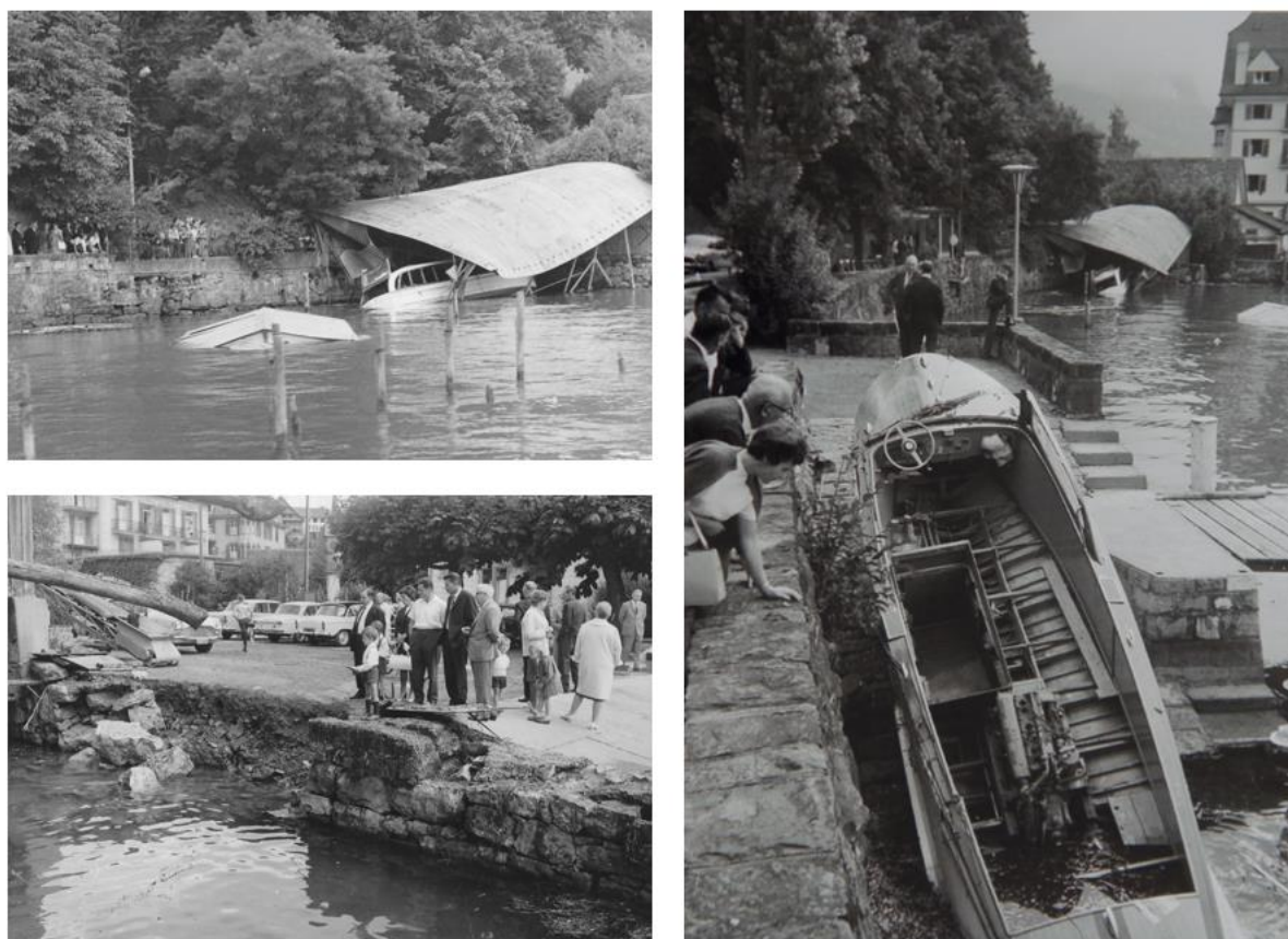
Fig. 3-4: Photographs documenting the damage and shore erosion (lower left image) caused by a rockfall-generated impulse wave at Weggis in 2.5 km distance on August 8, 1964 CE (photographs: historical archive Vitznau).
