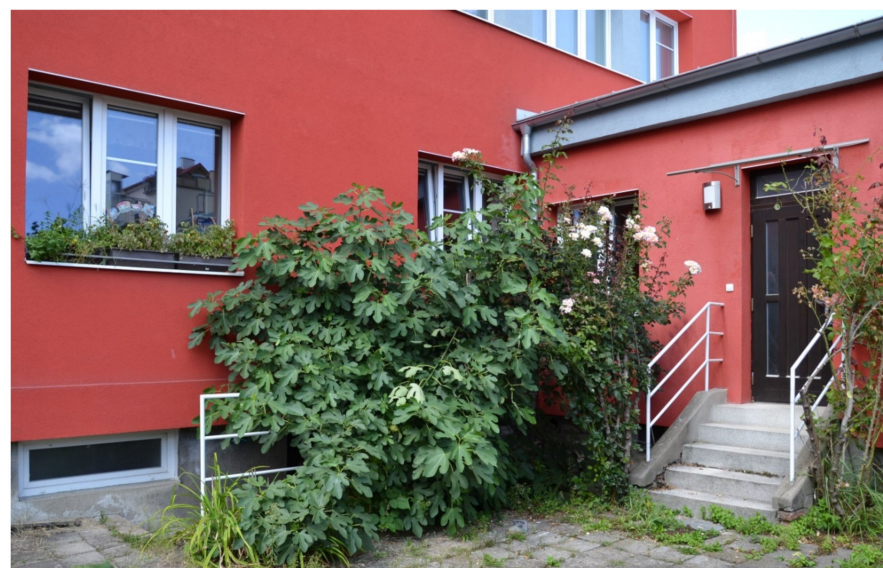
Figure 7. The fig tree and roses east of the building as part of the adaptation to global climate change. Author: Petr Klusáček.
