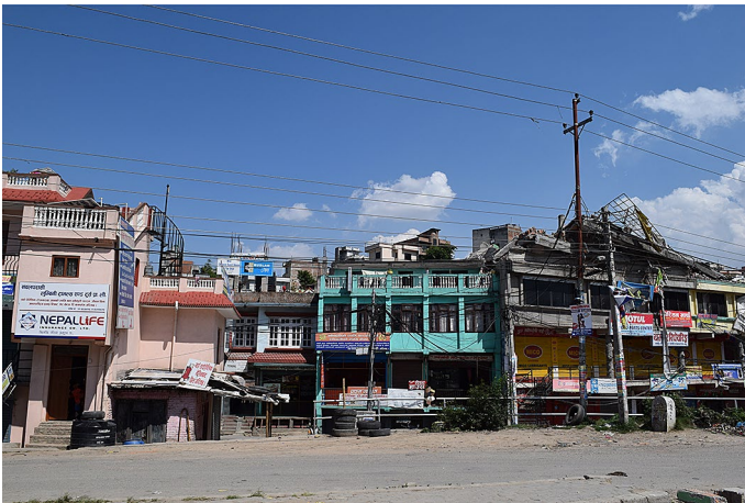
Fig. 15 Structural damage observed at Kalanki near Solti—no evidence of liquefaction (Liq. ID 10 in Table 6) [Photo: RM Pokhrel]
