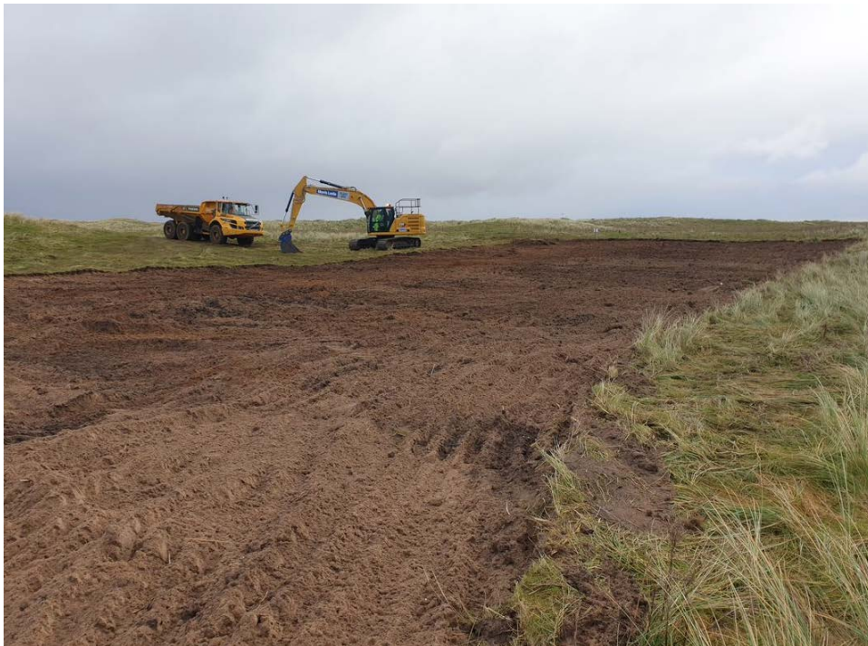
Figure 22. Turf stripped using heavy machinery at South Walney Nature Reserve, Jan 2021. Photo, Cumbria Wildlife Trust
