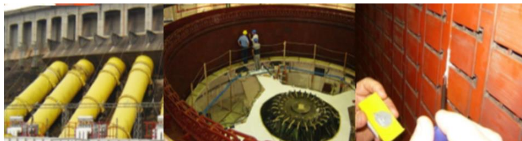
Fig 2.23: Implementation of FBGSs on a large hydroelectric power plant in Brazil [164]
