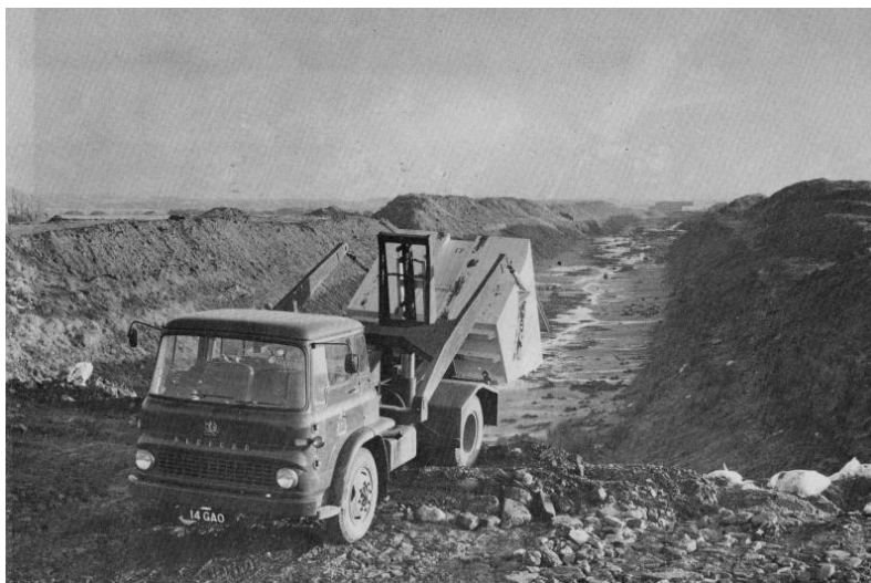
Figure 2. Operation of the LLWR trench disposal system in 1961. 6
