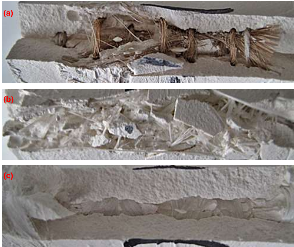
Figure 14 : Broken test specimens showing fractured surface of fibrous plaster under flexural loading. (a) Fibrous plaster with hessian reinforcement (b) Fibrous plaster with continuous fibreglass mat (CFM) reinforcement (c) Fibrous plaster with quadaxial glass fibre reinforcement
