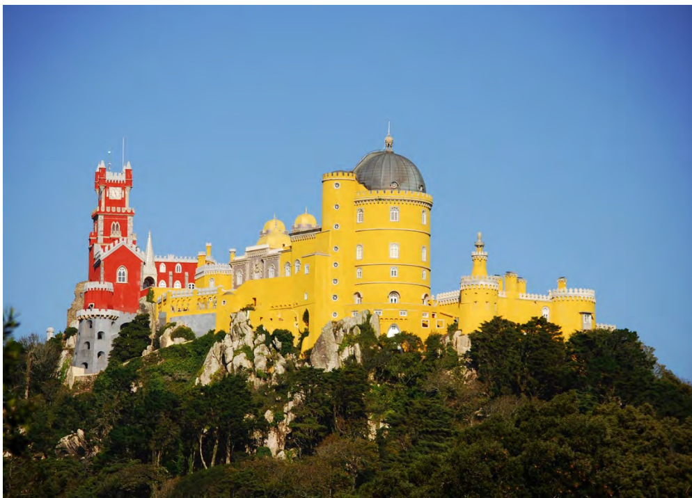
Fig. 1: Castellated Palace of Pena, Sintra. View from the southwest (photograph provided by the author).
