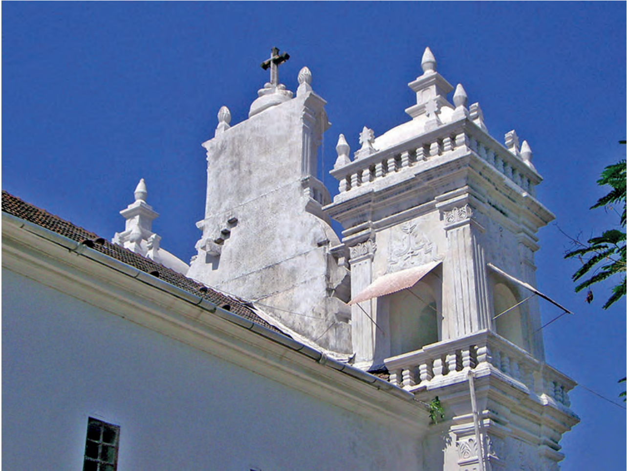
Fig. 4. View of the backside of the false dome, Church of Saint Stephen, in Juá Island, Goa, India. Photographed by the autor.
