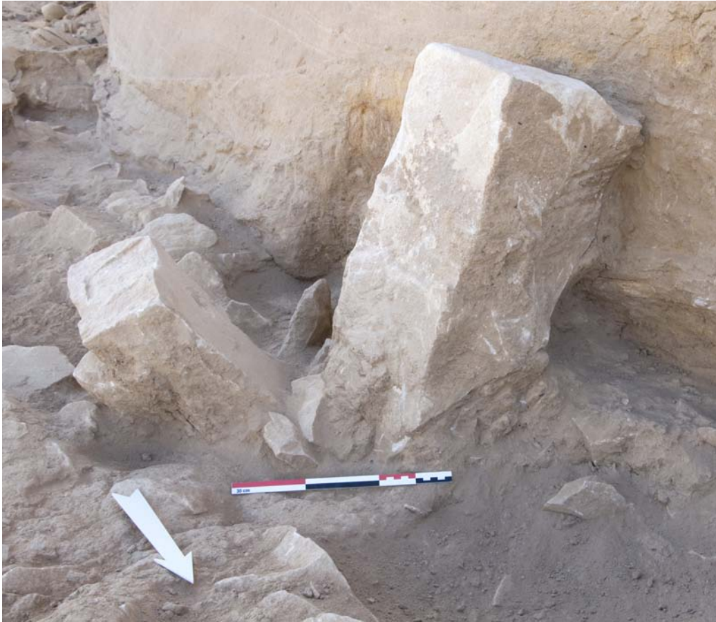
Fig. 69. Block which collapsed against the rock face
