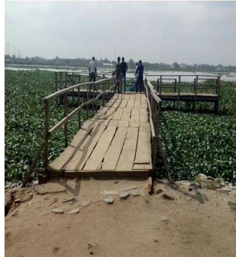
Figure A.5: Image of the loading bridge Source: Authors' Field work (2017)
