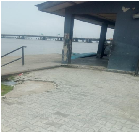
Figure A.15: View from the entrance showing the office right wing section Source: Authors' Field work (2017)
