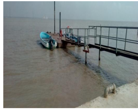
Figure A.12: Ramp access to floating platform Source: Authors' Field work (2017)
