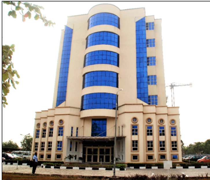
Figure 1: Covenant University Senate Building Façade
