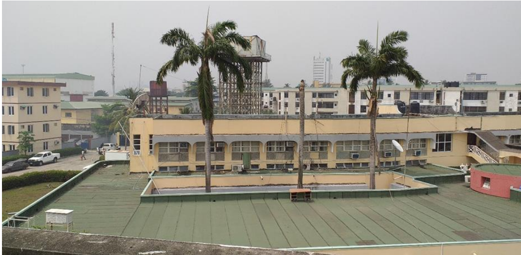
Fig 2.5: Presence of courtyard in the Nigerian Institute for Oceanography and Marine Research building
