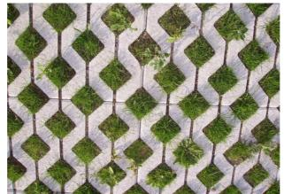
Plate 2.3: Sustainable Drainage – Permeable Pavement Sidewalks and Gardens Source: [18].
