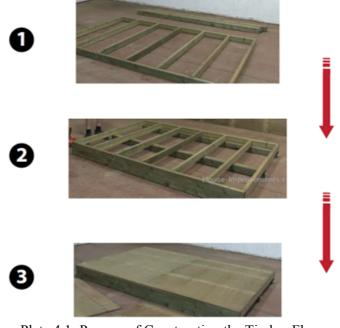
Plate 4.1: Process of Constructing the Timber Floor Source: [20].
