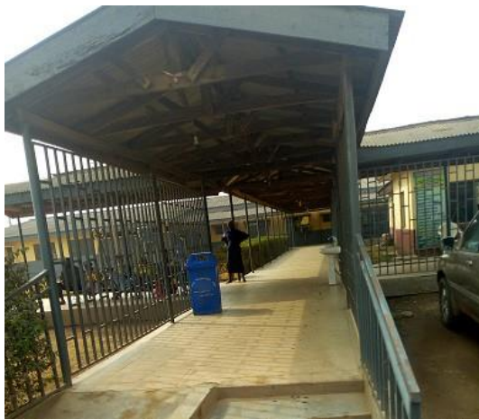
Plate 1: A Walkway on Site
