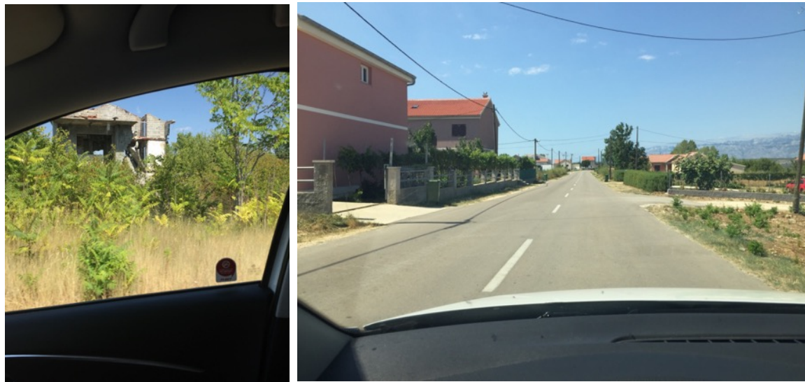
Left: A ruined home in Islam Grčki, 7 August 2017. Right: A re-paved road with fully reconstructed homes in neighbouring Islam Latinski, 7 August 2017.
