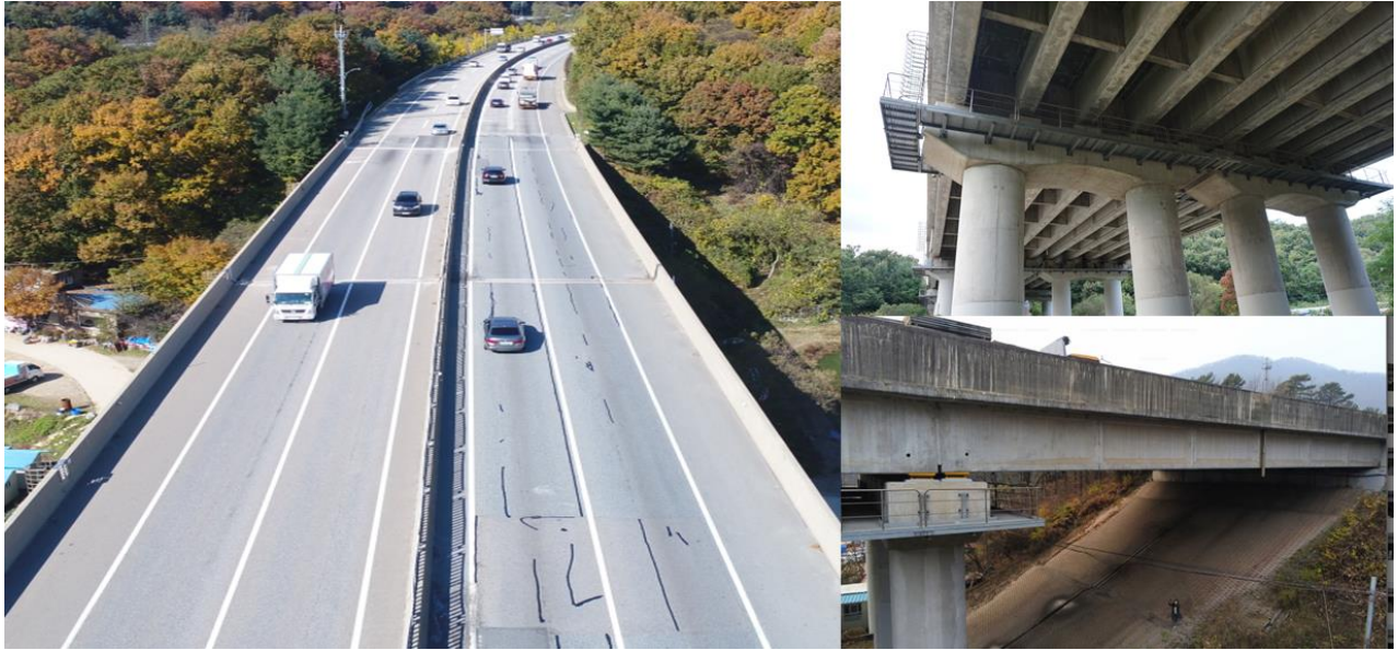
Figure 3. Case study bridge
