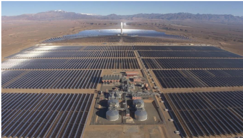
Figure 1.2: Solar PV power plant [7].
