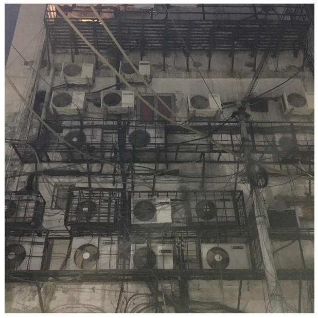
Figure 27: The exhaust sections of air conditioners at the back of a building in an affluent market neighbourhood in south Delhi. Photograph from July 2018, taken by author
