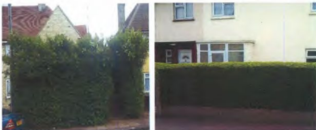
Figure 5.16 Extract from LISP proforma showing overgrown hedgerows
