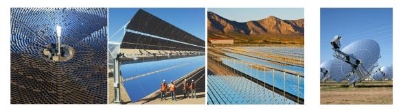
**Figure 2.3:** Some examples of solar field and solar collector configurations (from left to right): solar tower (courtesy: Solar Reserve), parabolic trough [101], linear Fresnel (courtesy: Novatec Solar) and solar dish (courtesy: Tessera solar).
