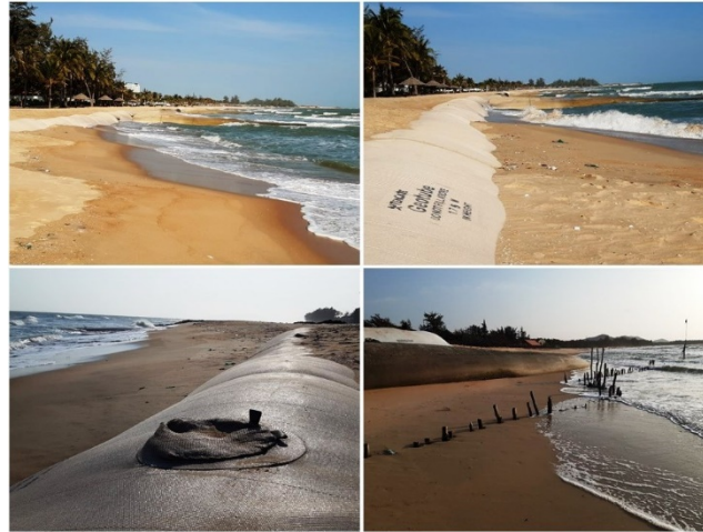
211 Figure 3: Soft measures using Geotubes in Ba Ria-Vung Tau, southern Vietnam
