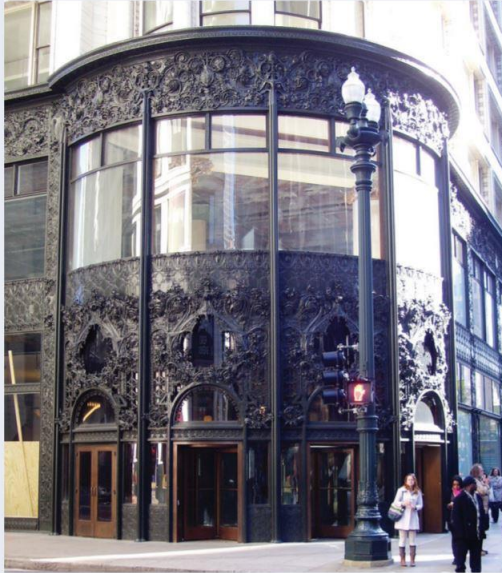
Figure 7.35 | The northwest entrance to the Carson, Pirie, Scott and Company Building
