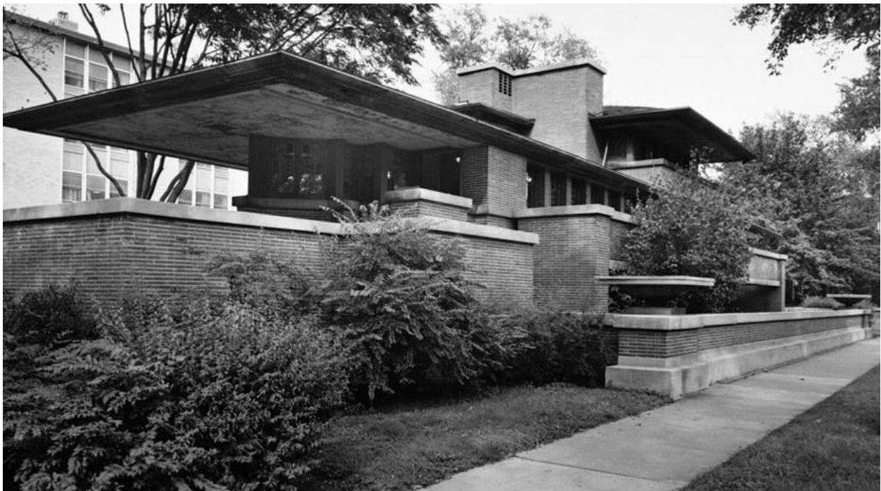
Historic American Buildings Survey Cervin Robinson, Photographer, 18 August 1963 EXTERIOR FROM SOUTHWEST - Frederick C. Robie House, 5757 Woodlawn Avenue, Chicago, Cook County, IL 5 x 7 inches (Library of Congress HABS ILL,16-CHIG,33--3) CC0.
