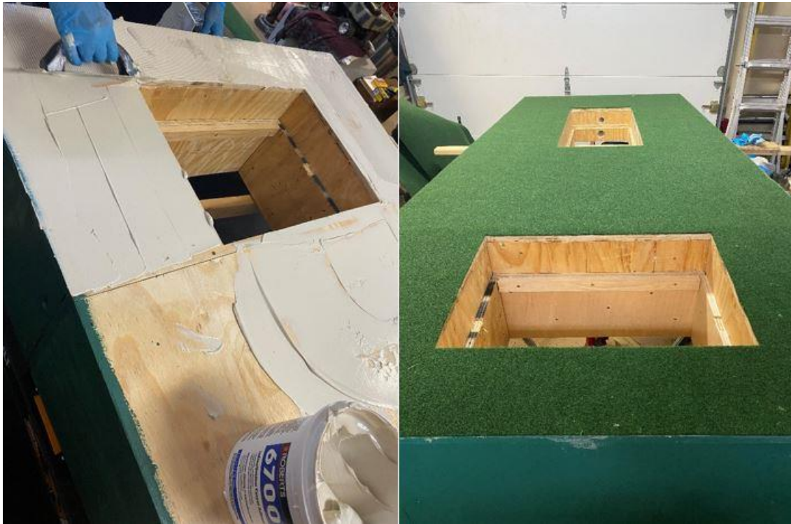
Figure 6. Surfacing the mound with artificial turf. The mound was surfaced with artificial turf and attached using artificial turf adhesive. The turf had a low nap and provided optimal traction.
