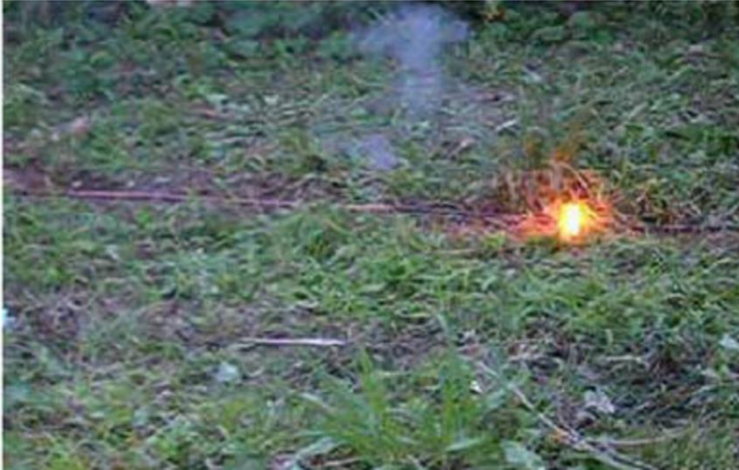
Figure 4.1 A downed conductor arcs to the wet grass [76, 77]
