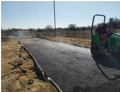
c) Compaction of HMA layer.
