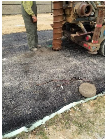
(a) Drilling Sensor Hole
