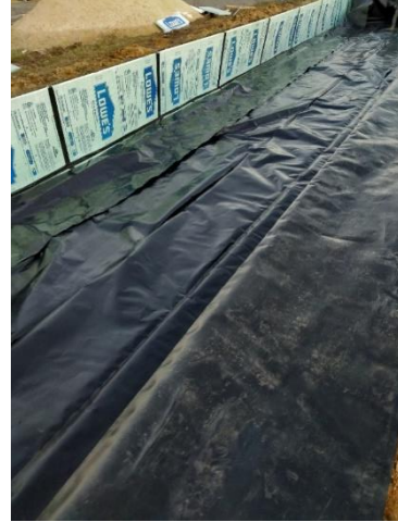
(b) Impermeable Membrane
