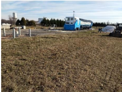
(a) Marking Perimeter
