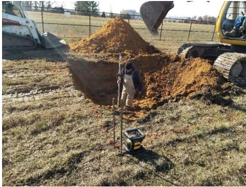
(c) Depth Check when Excavating
