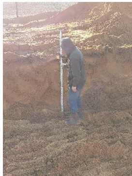
(c) Depth Check when Excavating
