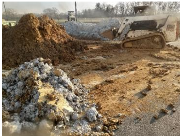
Blending of Soils Using a Bucket Loader
