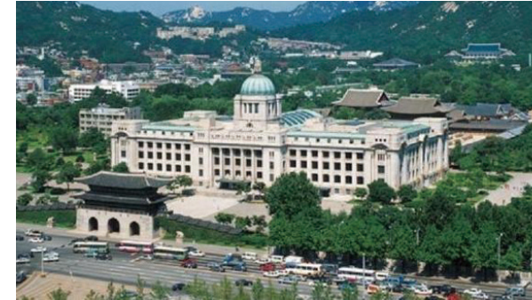
Before the demolition
