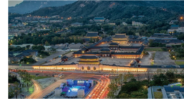
After the demolition
