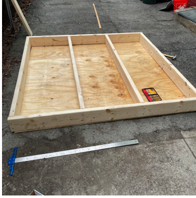
Building the platform.
