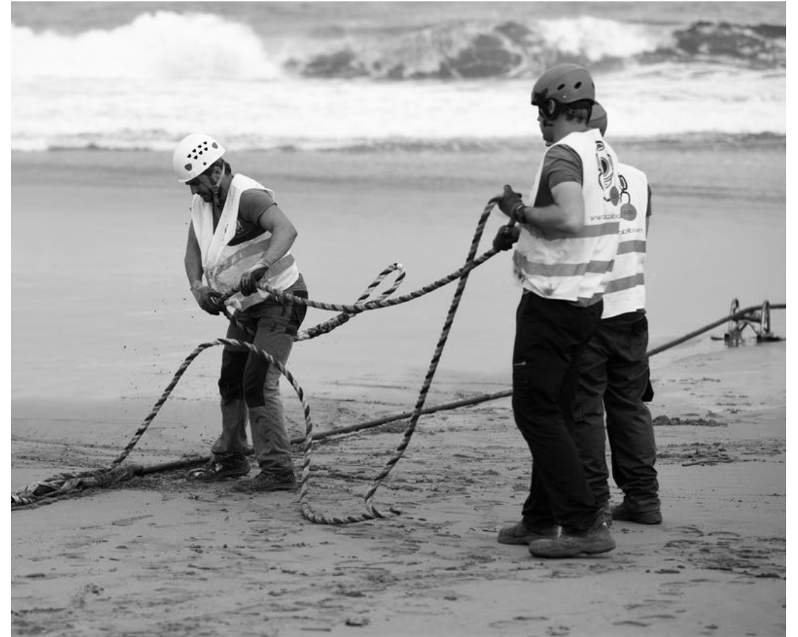
Deep-sea fiber optic cables being pulled out of the water. / AFP
