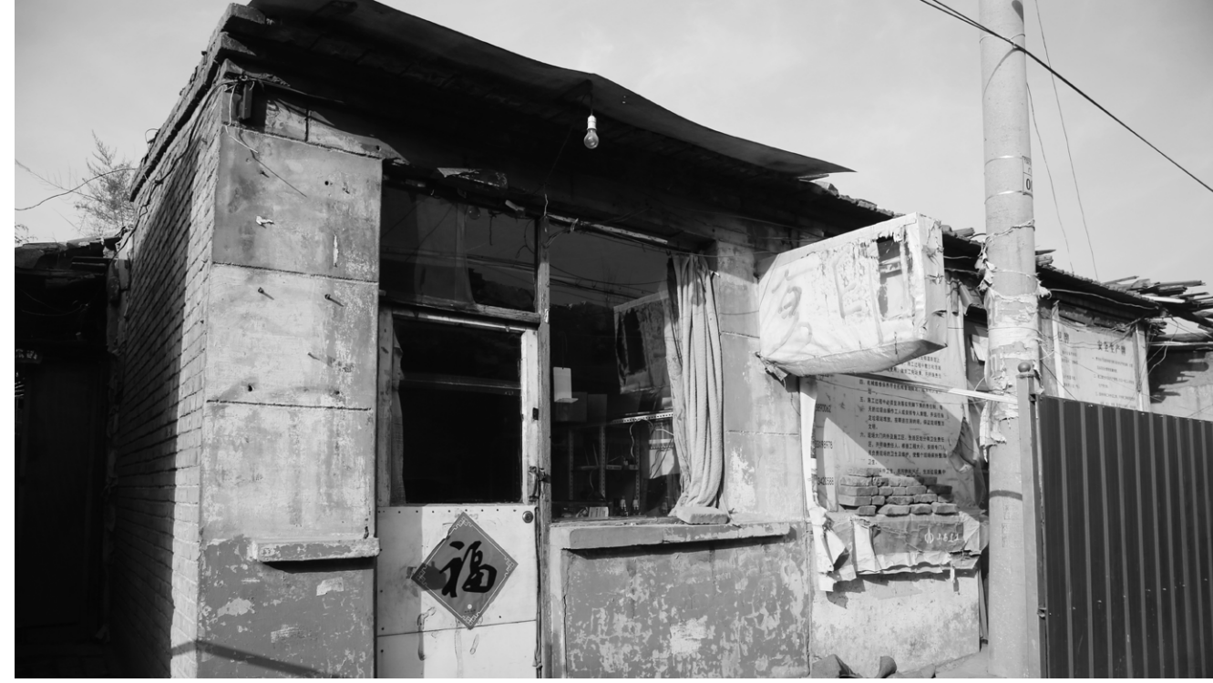
A print shop in the old town, which is one of the few public facilities
