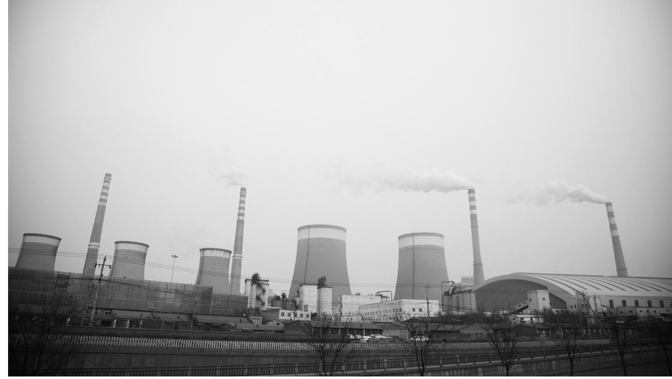
Largest power plant in Datong
