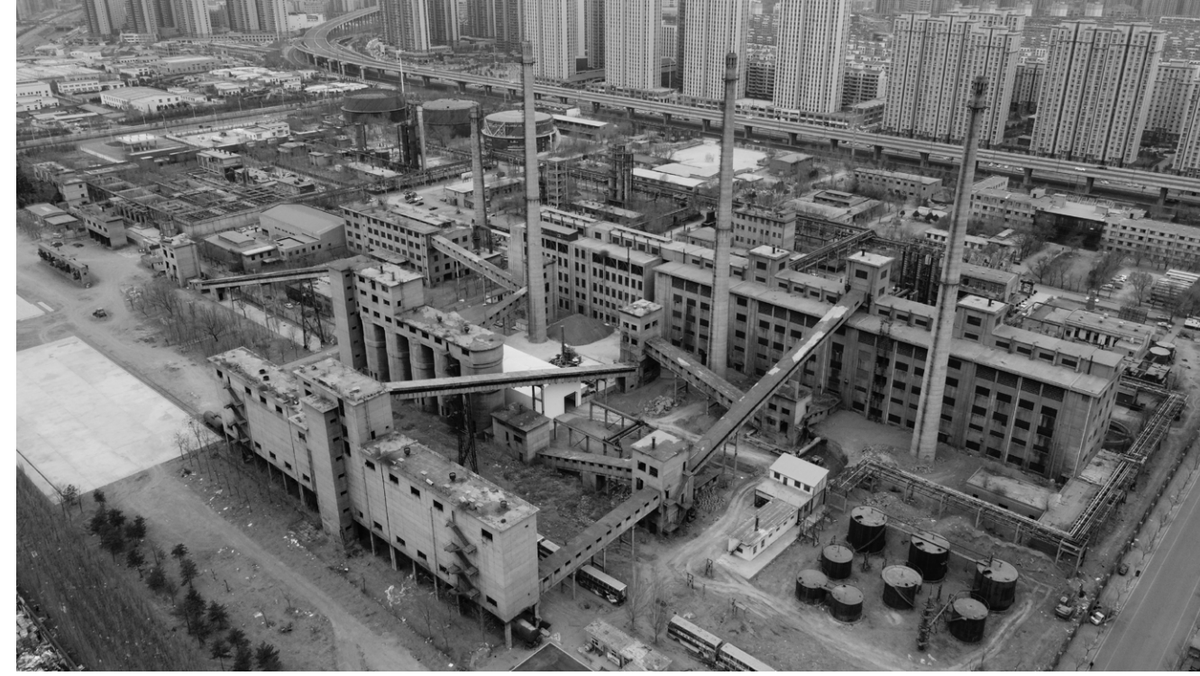
Abandoned factory exterior
