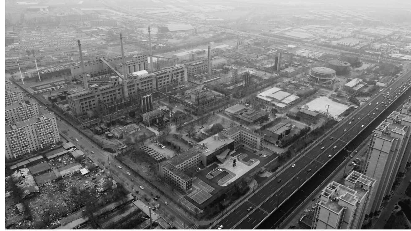
Coal gas factory, drone aerial view
