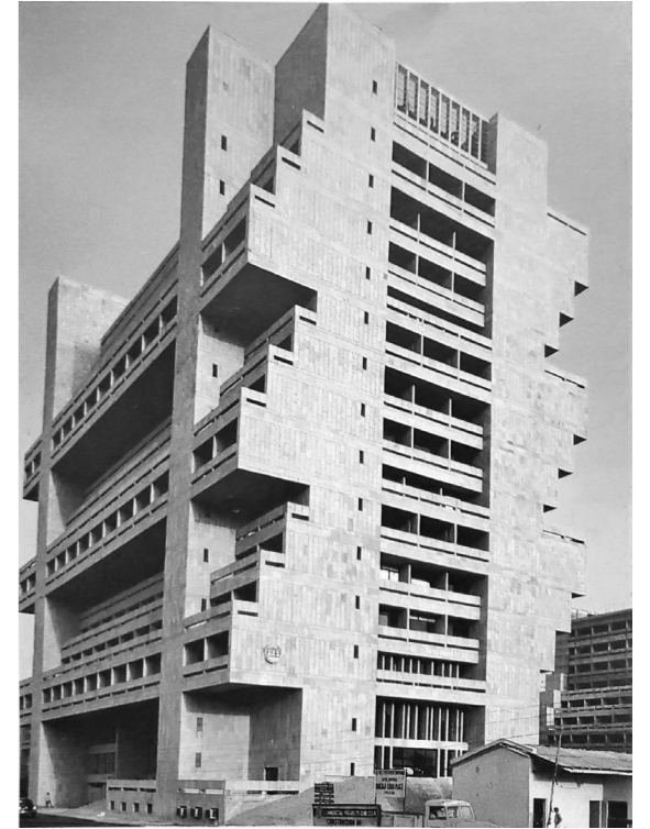
East facade of Engineer India house in Bhikaji Cama office complex built by Raj Rewal.
