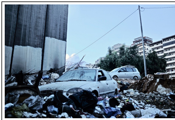
Figure 6. Wall, rubbish and new housing construction in Ras Khamis (Shuafat Refugee Camp area), October 2017.
