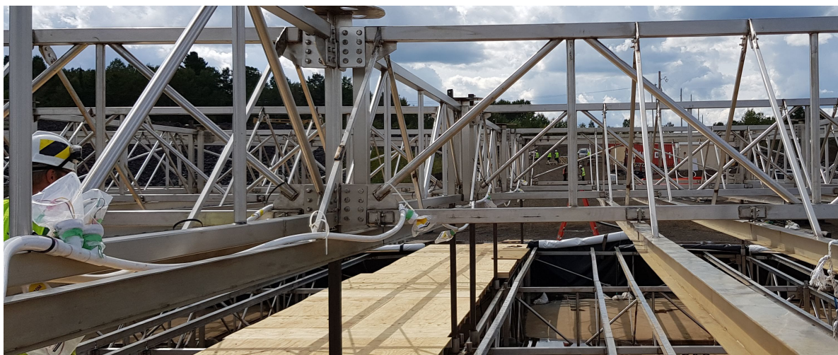
Figure 4.9: Picture of a Nikhef POM to Nikhef-container manifold (in white) attached to the top-cap of the CHIPS-5 detector. In the left of the image, two unattached Nikhef POM pigtail connections are seen, both covered in green tape and a plastic bag. The manifolds can also be seen in the graphical rendering of the top-cap shown in Figure 3.17.
