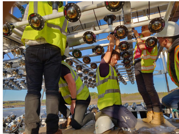
(b) POM installation.
