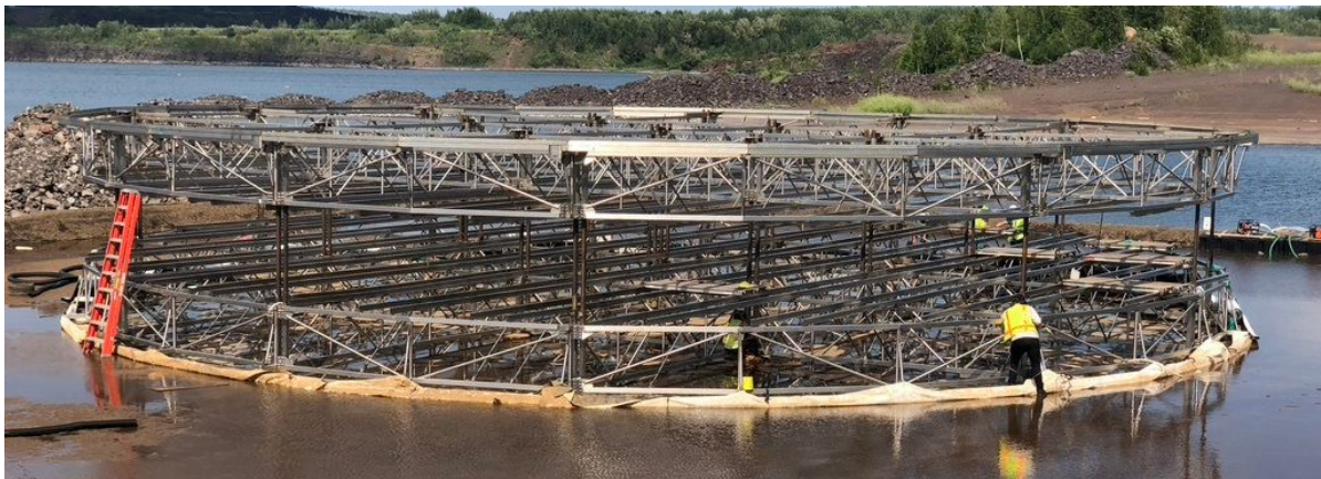
Figure 3.11: Picture of the CHIPS-5 structural frame with humans for scale. The endcaps can be seen separated by steel struts. Rows of stainless steel stringers are attached to the inside of each endcap for instrumentation mounting.
