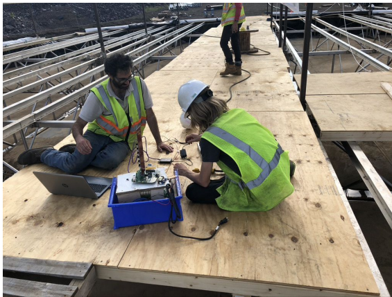
(a) Connection testing.
