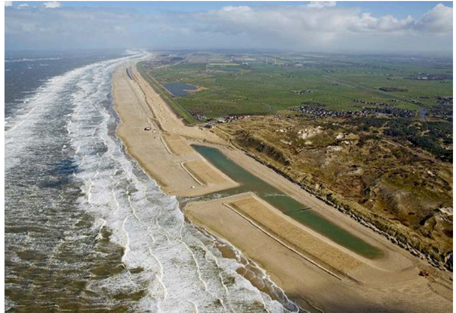
Figure 1 | The Hondsbossche Dunes in the Netherlands, a soft natural barrier reinforcing a local sea dike.
