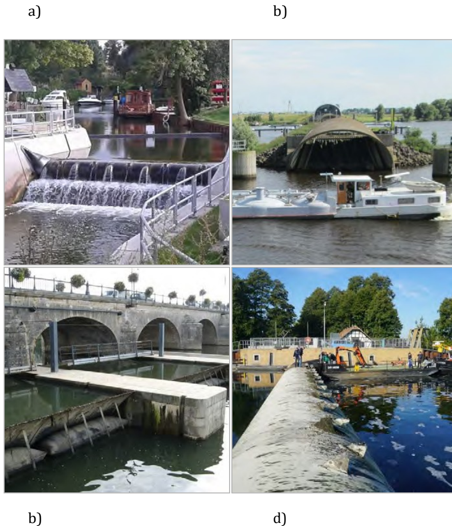
Figure 2: Applications of inflatable gates at waterways
