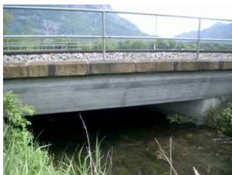
Fig. 8: Culvert through the railway dike [6]
