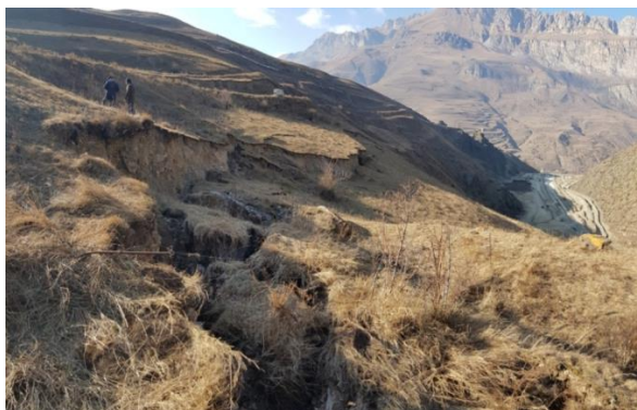
Fig. 1. Wall of landslide separation caused by cutting of the lower part of the slope during the liquidation of Fiagdón tailing dump, photo: December 2019
