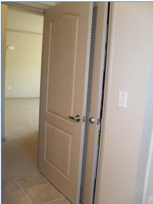
Figure 4.7: Unit-Type C1 Mechanical Closet and Hall Bathroom Doors
