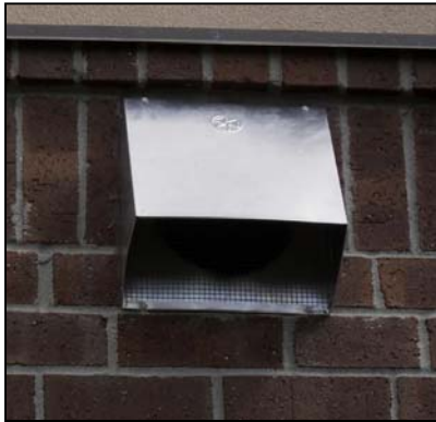
Figure 4.1: Metal Wall Cap on Test Building
