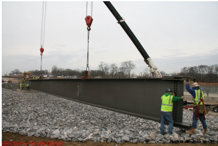
Figure 33: Holding of Girder 105A1 by the 175-ton and 40-ton cranes
