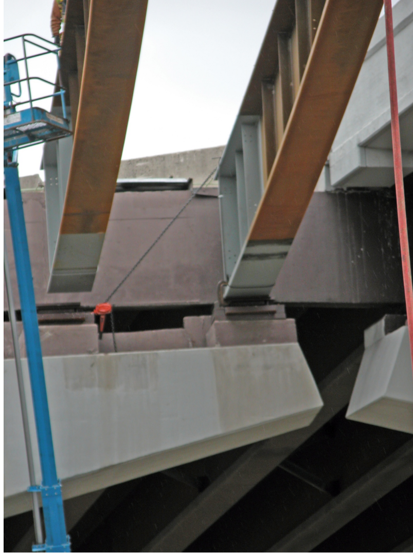
Figure 62: View of come along on girder 175A15
