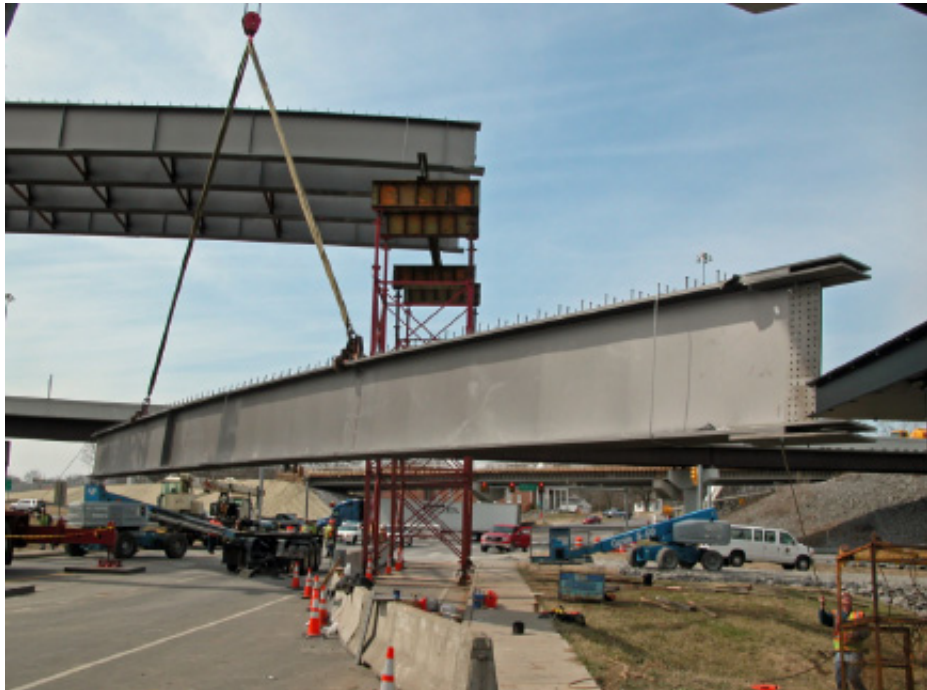
Figure 87: Girder 170A14 being lifted
