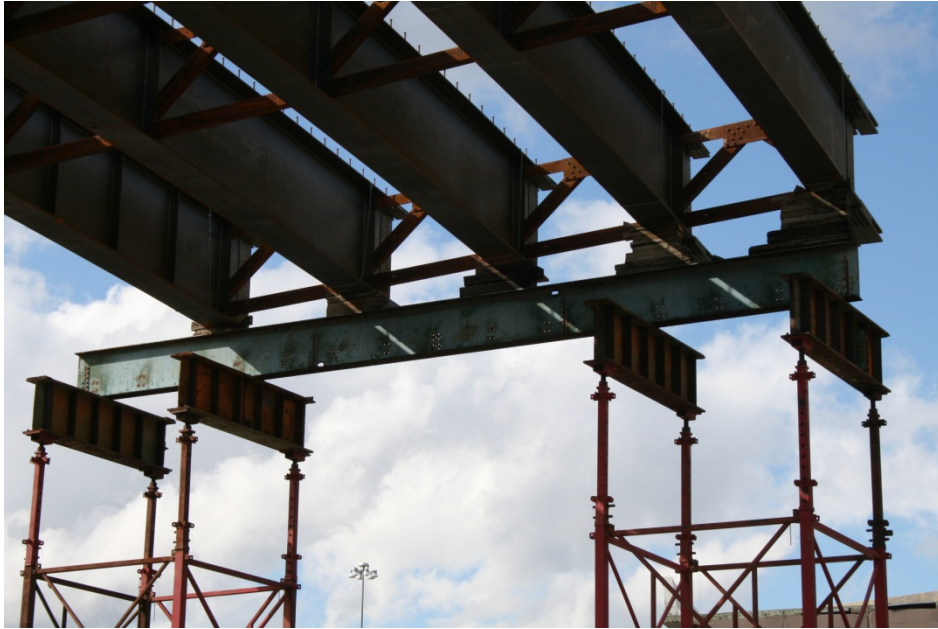
Figure 59: Cribbing Placed Between Top of Shoring Tower and Bottom of Girders
