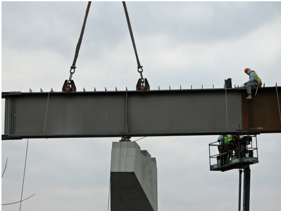
Figure 54: Splicing of Girders 131E7 and 136E8
