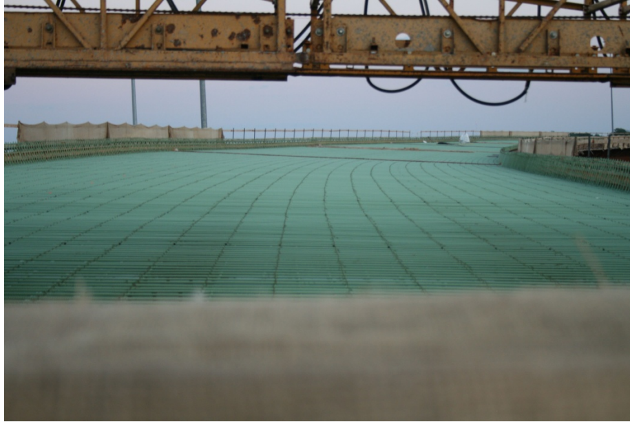
Figure 71: Reinforcing and screed in place, awaiting concrete
