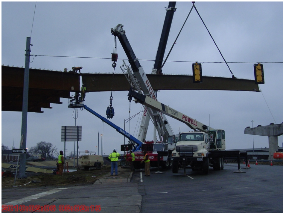
Figure 48: Positioning of Girder 125A5
