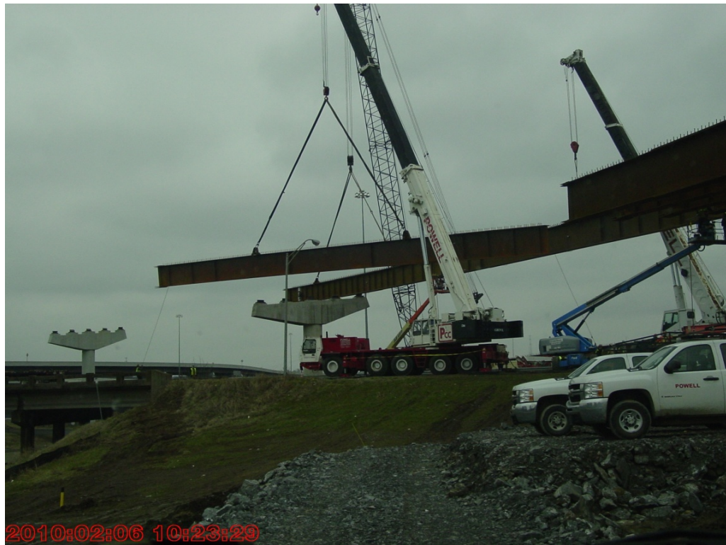
Figure 51: Positioning of Girder 124B5
