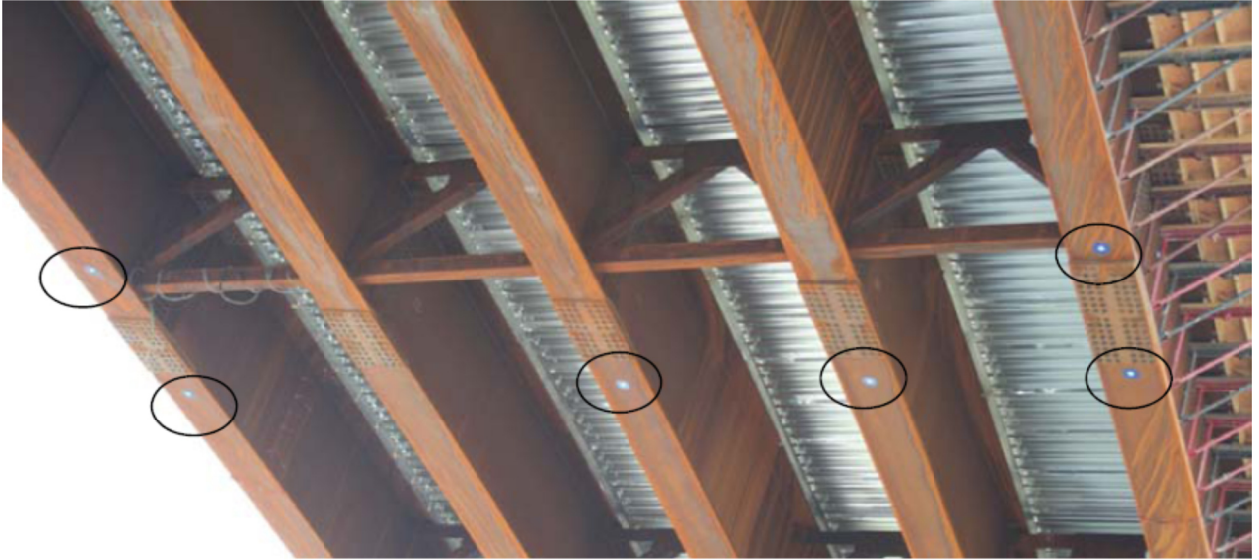
Figure 28: Underside of bridge showing reflective targets attached to bottom flanges
