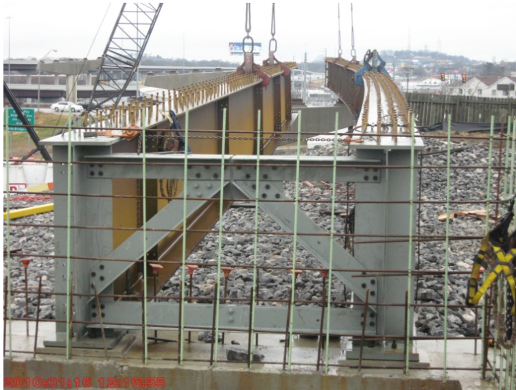
Figure 37: One Cross Frame Attached Between Girders 104B1 and 105A1
