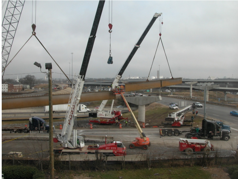
Figure 43: Positioning of girder 120A4 in Preparation for Splicing to Girder 115A3
