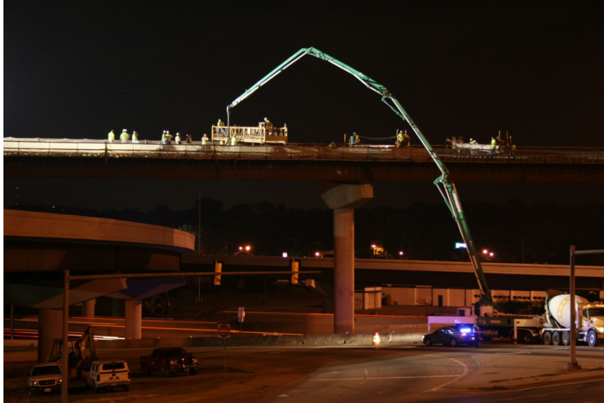
Figure 72: Concrete placement during coolest part of the day
