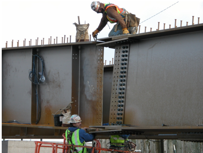
Figure 40: Workers Splicing Girders 109B2 and 110B1
