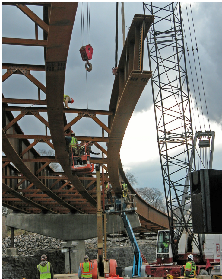
Figure 47: Installation of cross-frames between Girders 117D4 and 116E4
