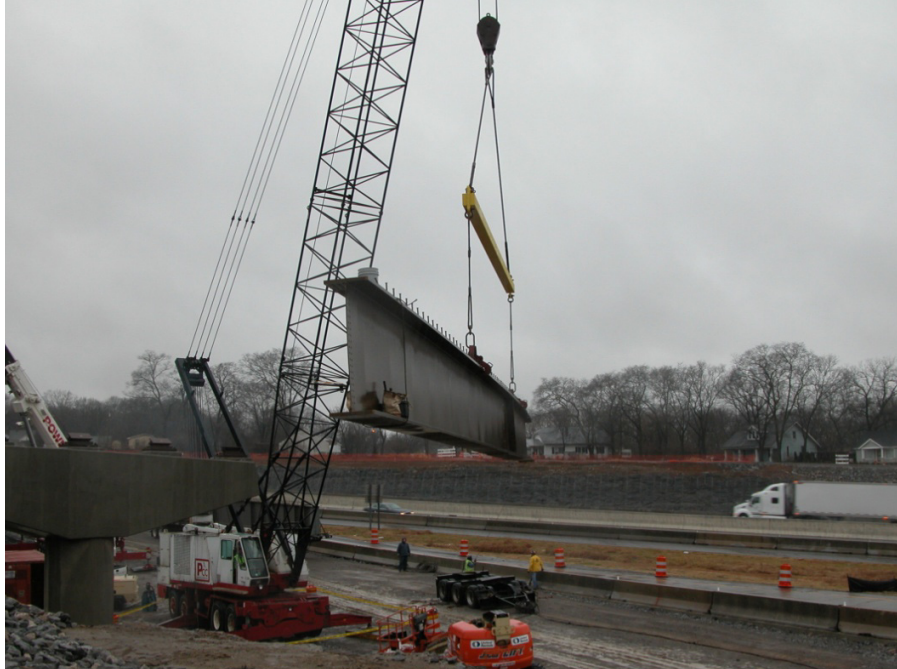
Figure 34: Lifting of Girder 110A2
