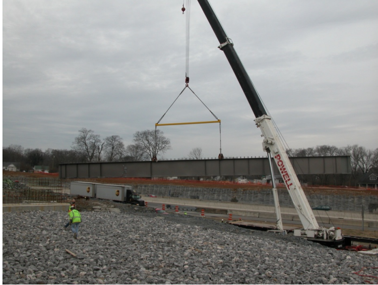
Figure 32: Lifting of Girder 105A1
