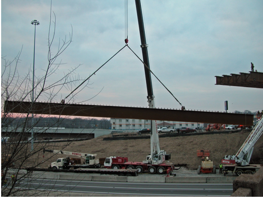
Figure 53: Lifting of Girder 131E7
