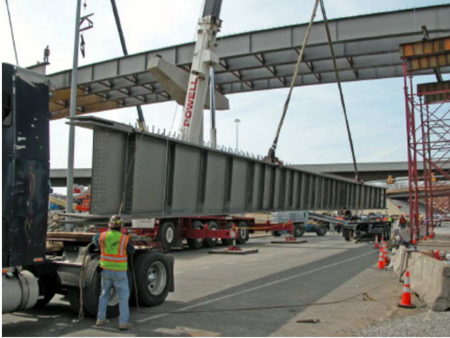
Figure 86: Girder 170A14 being lifted
