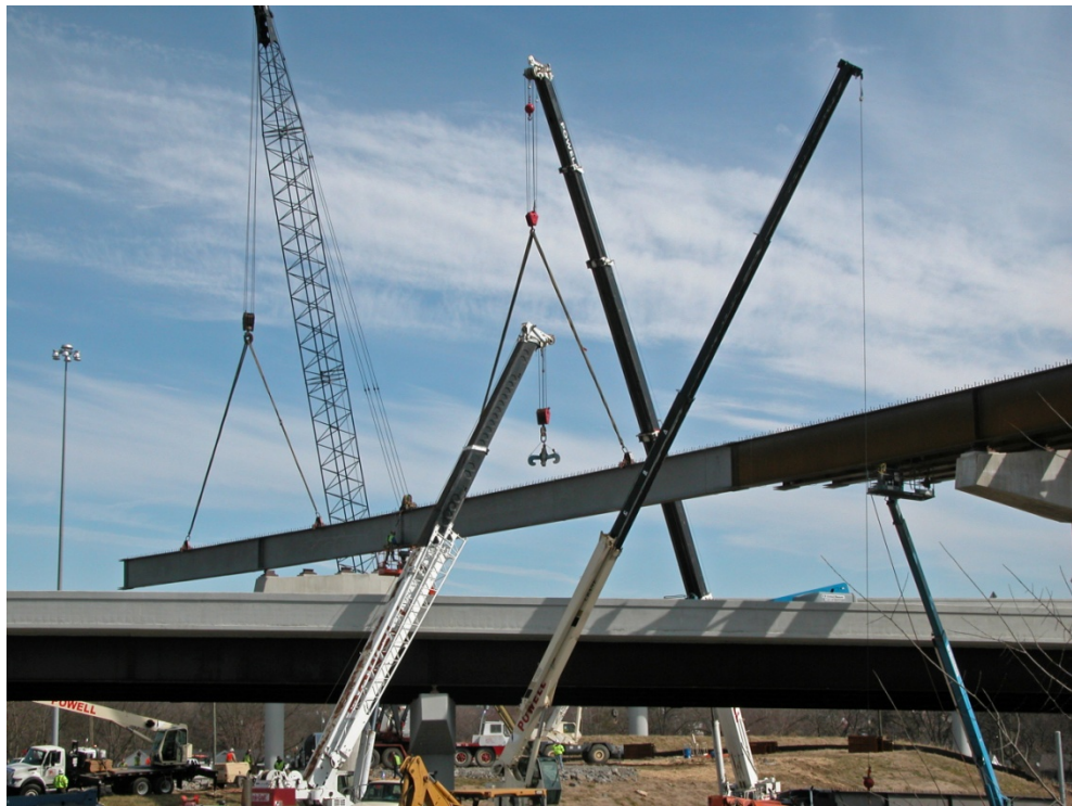
Figure 56: Connection of Girder 156E12 to Girder 151E11
