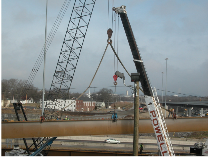
Figure 44: 150-ton Lattice Boom Lifting Crane Being Released from Girder 115A3
