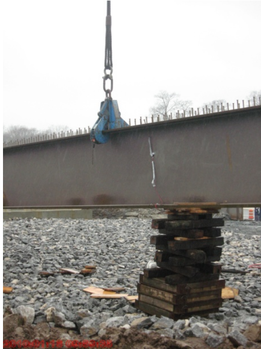
Figure 36: Cribbing under Girder 105A1
