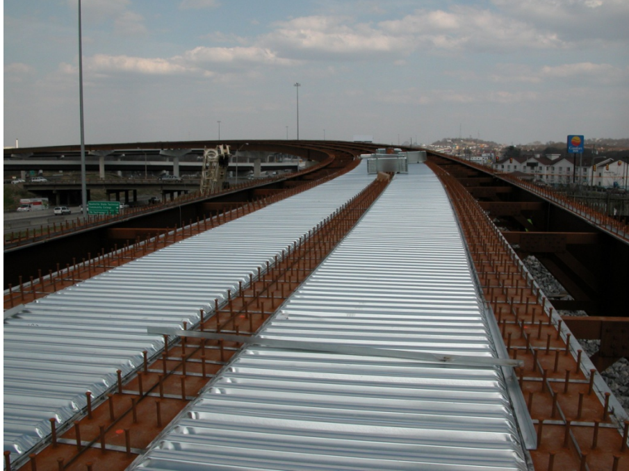
Figure 69: Metal decking partially installed
