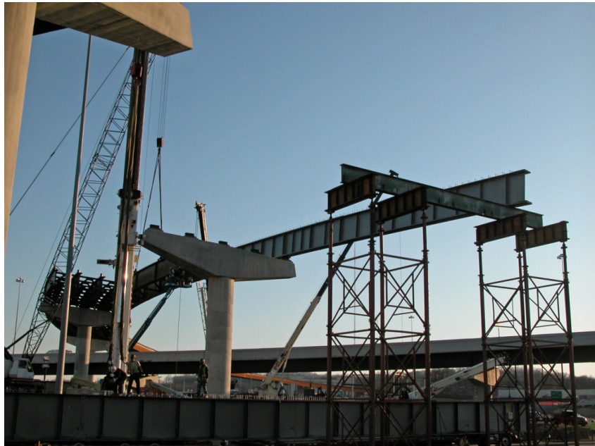
Figure 57: View of Shoring Tower after Placement of Girder 162D13
