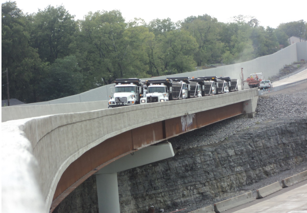
Figure 3: View (Looking West) of Ramp B during Load Testing
