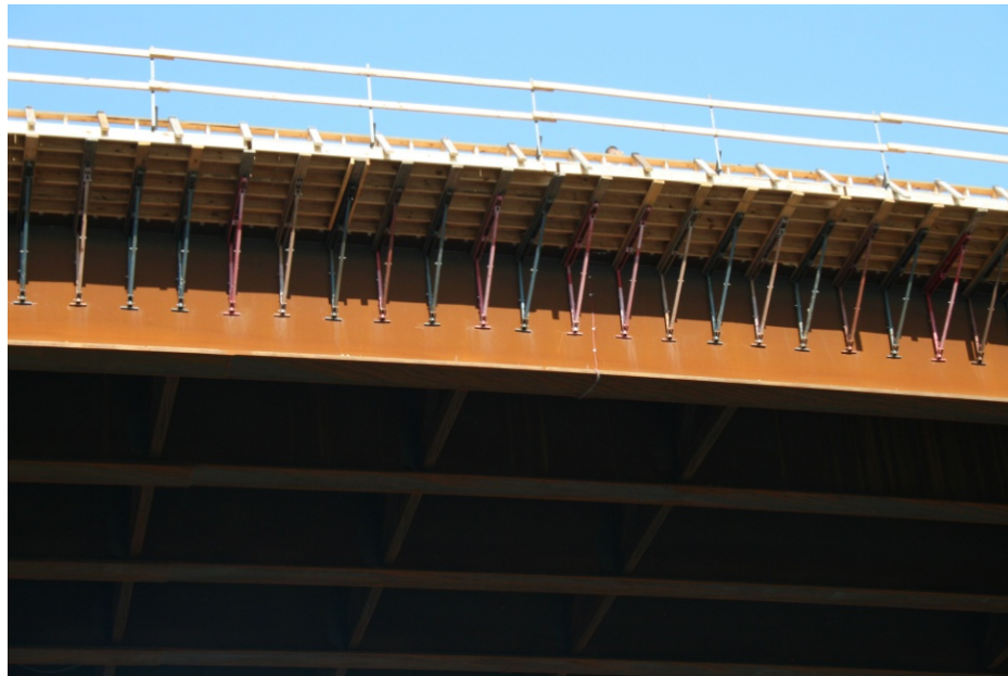
Figure 70: Concrete formwork supported by overhang brackets
