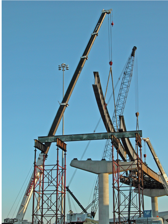
Figure 58: Lifting of Girder 167D14
