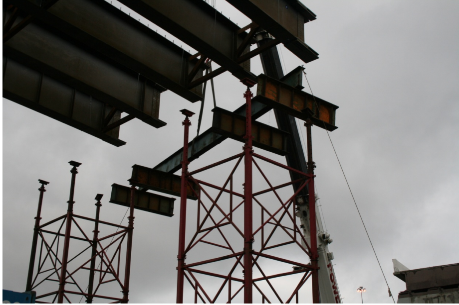
Figure 60: Shoring tower at span 7 after removal of cribbing
