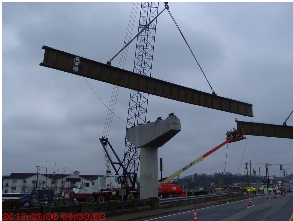
Figure 49: Positioning of Girder 130A6
