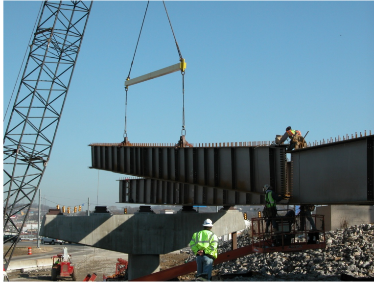
Figure 41: Placement of Girder 108C2
