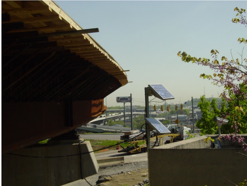
Figure 27: Installation of solar panels at Bent No. 2
