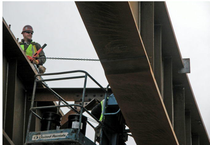
Figure 45: Use of a come-along between girders 120A4 and 119B4 near Bent 1
