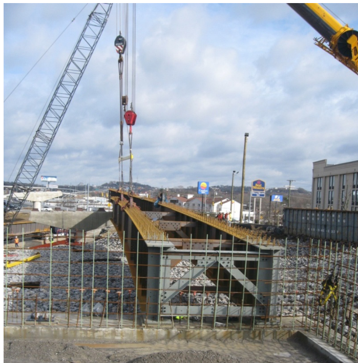
Figure 38: All Cross-Frames Attached Between Girders 104B1 and 105A1.
