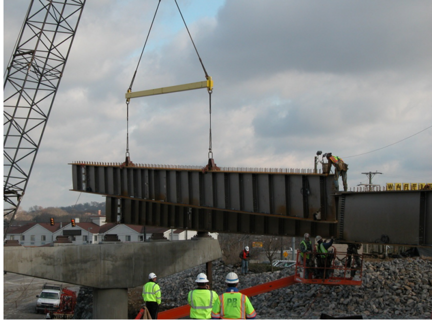
Figure 39: Lifting of Girder 109B2
